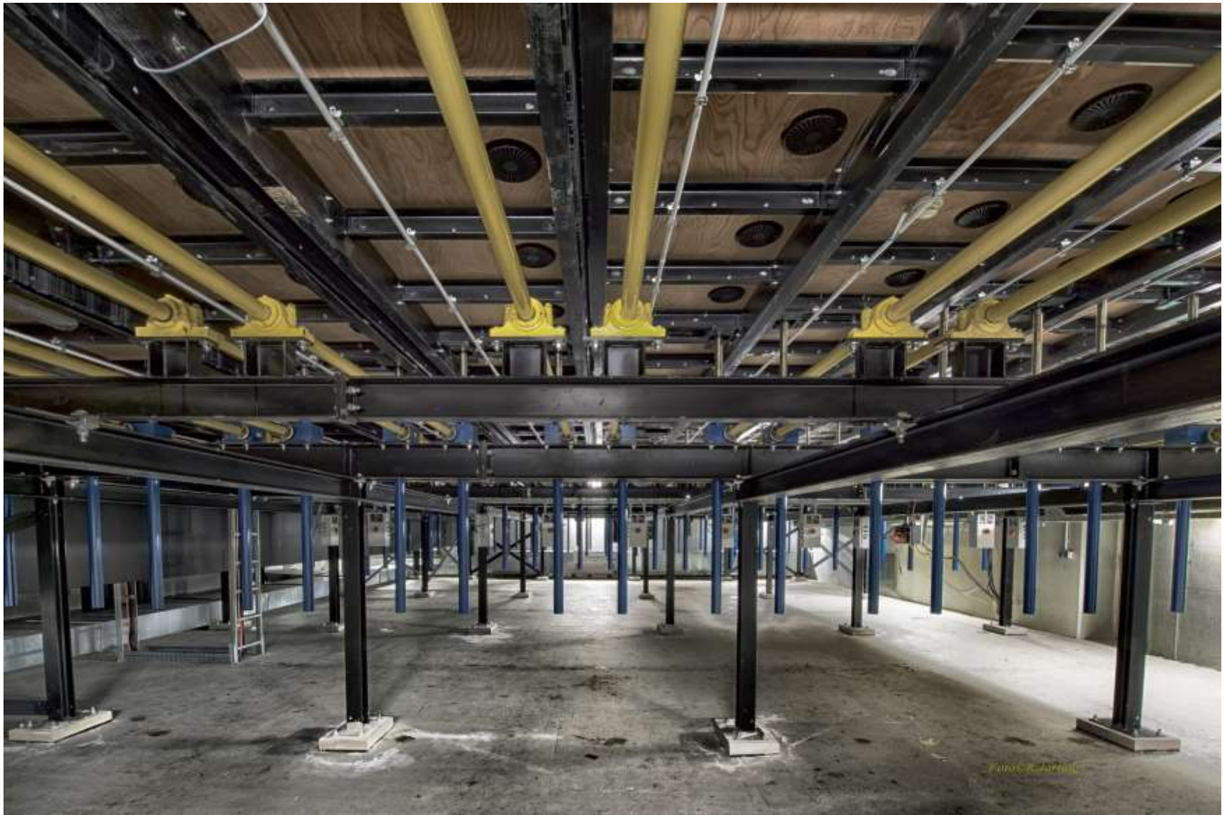
2021-02-18-rj-2-Ralf Jarling- Vogtlandhalle-DSC_5435
